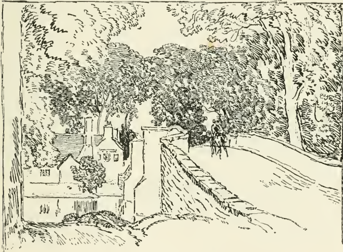
Eamont Bridge, near Penrith.
